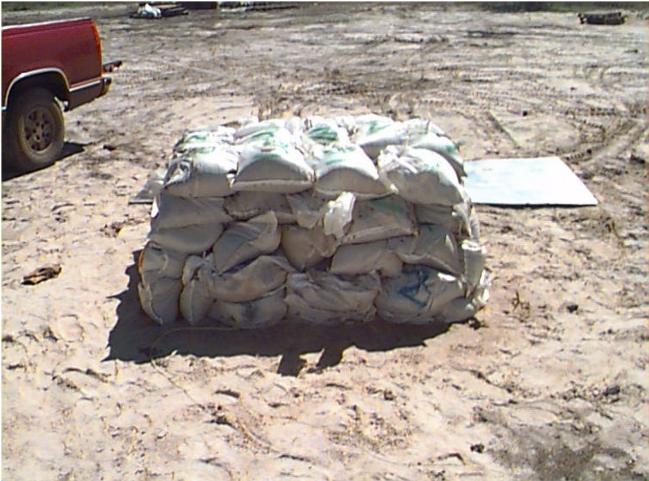
FIGURE 3-3: SIDE VIEW – SANDBAG ENCLOSURE
